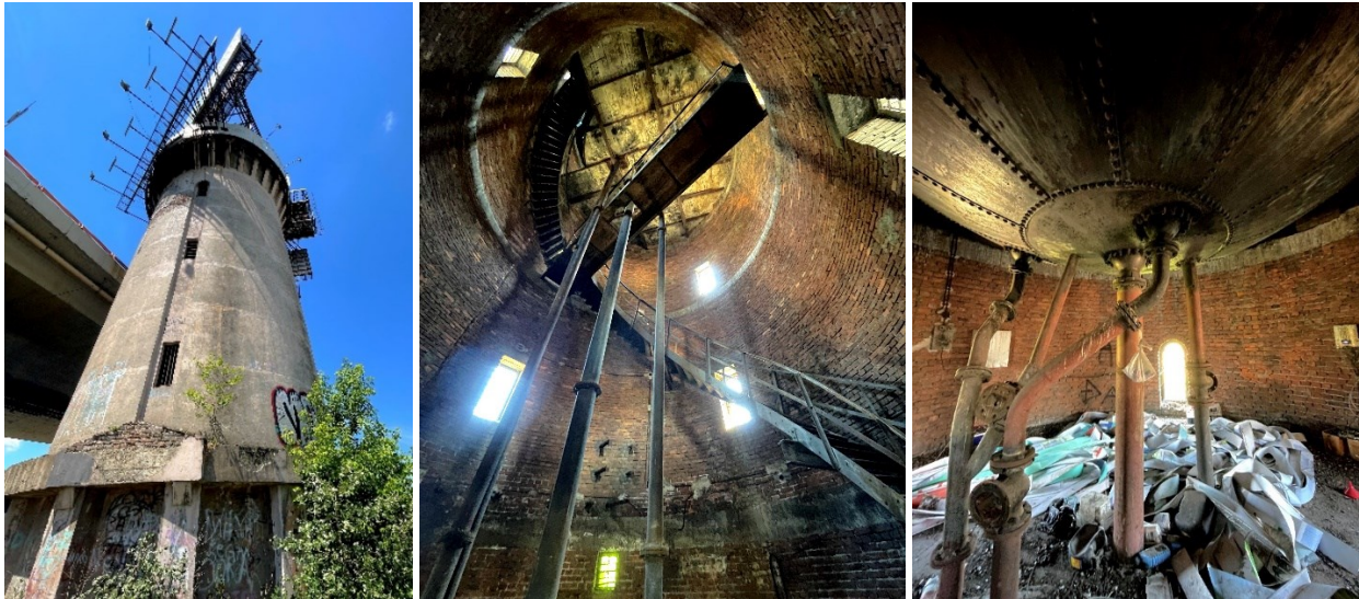
Figure 33, 34 and 35. The current state of the Vodotoranj
