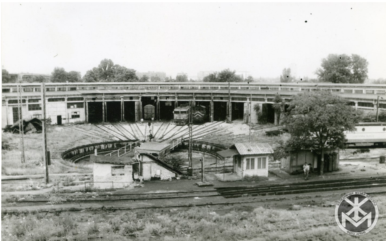
Figure 15. View of the central part of the semicircular hall of the Ložionica Belgrade - Belgrade Railway Station Complex (photographed by G. Matijević, June 1995, F.F.15 / 95). Railway Museum.
