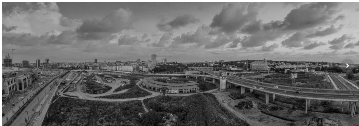
Figure 36. View of the Ložionica area
