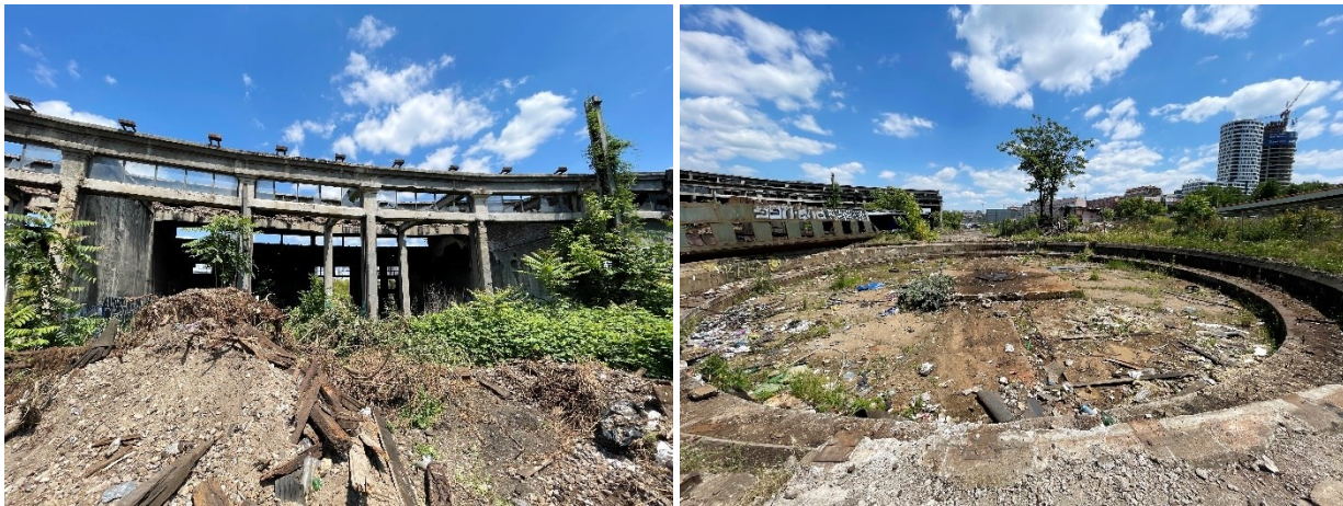
Figure 31 . and 32. The current state of the Ložionica and Okretnica complex
